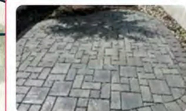
Permeable paving will help rainwater soak back into the ground and not lie on the surface.
